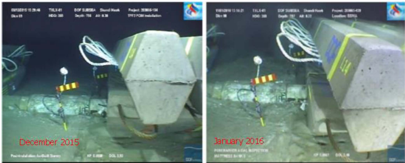
Figure 15—Flags with ruler markings installed adjacent to PCMs to facilitate displacement measurement
