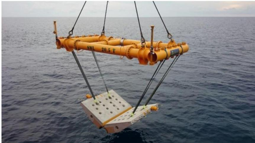
*PCM lifted Flat to minimise load transfer induced embedment.*
