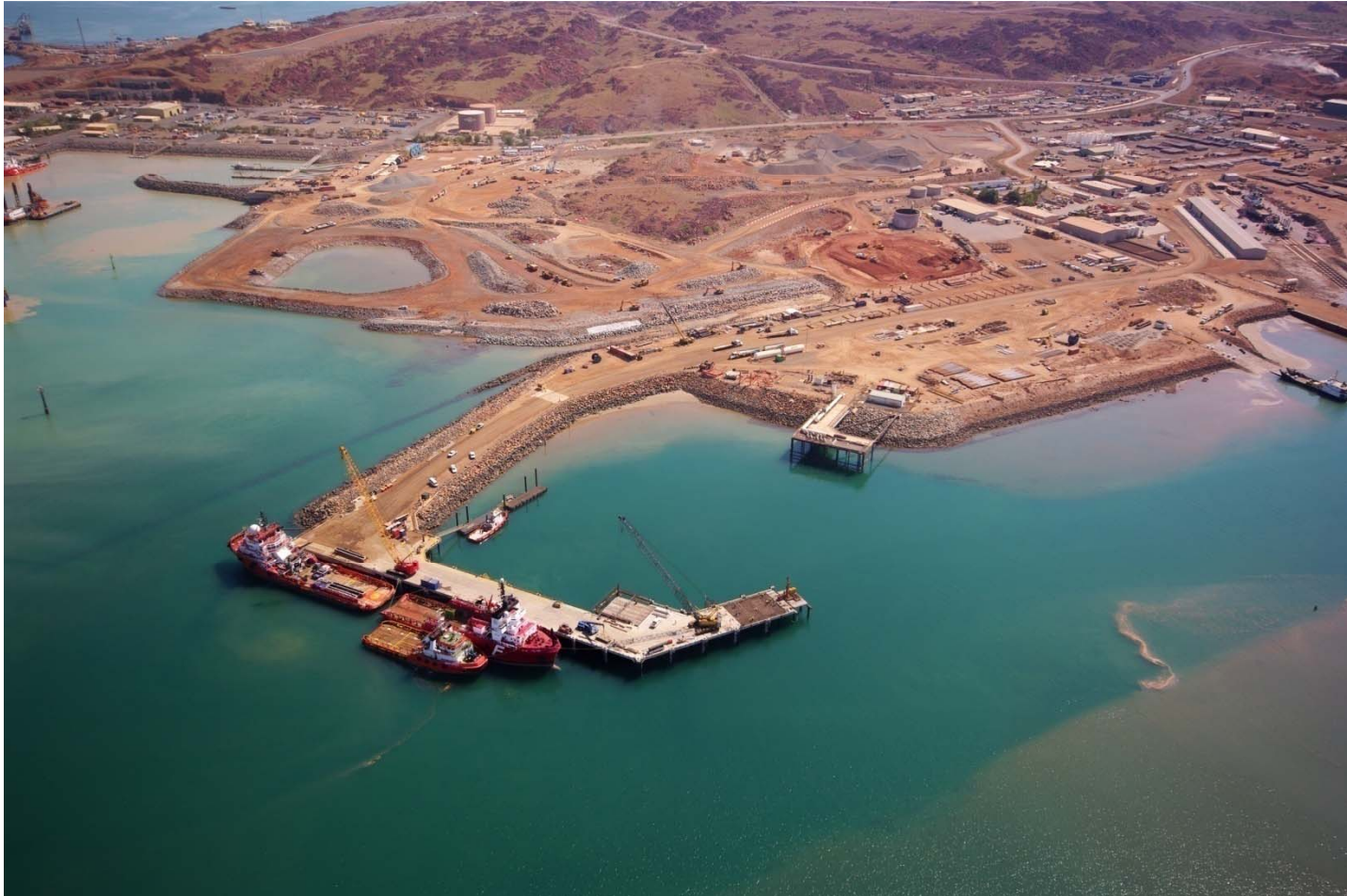
Mermaid Marine Supply Base, Slipway & Wharf
