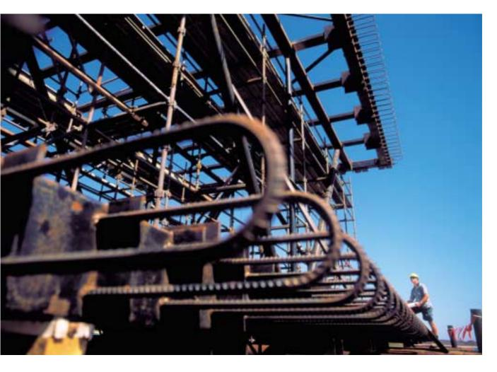
Shell of the first fabricated steel cell to be used in construction of the wharf.
