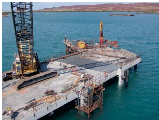
Extension to Dampier Supply Base wharf under way.
