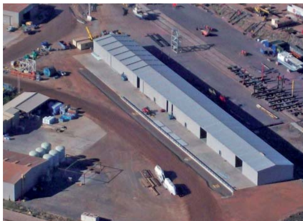
New 2,250m 2 warehouse at the Dampier Supply Base.
