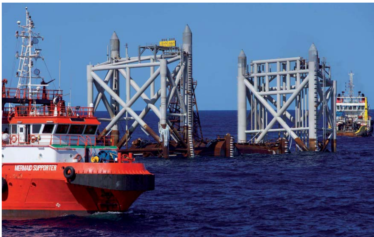
Woodside Energy's Angel Project jacket installation.
